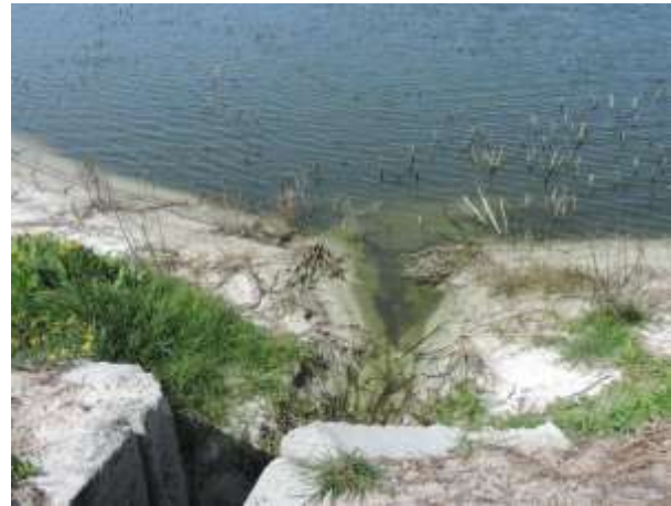
Trenches dug at two of the four outlet weirs of the pans at Strandfontein Section which were opened to assist the movement of water from the pans and into the adjoining canals (Photos: E. Essig 2016)
