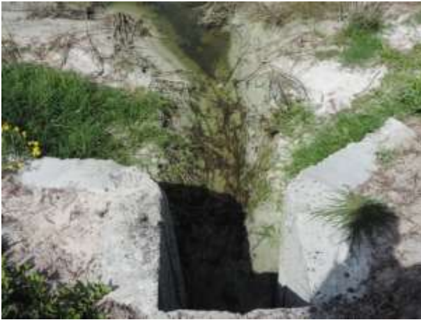
Trenches dug at two of the four outlet weirs of the pans at Strandfontein Section which were opened to assist the movement of water from the pans and into the adjoining canals (Photos: E. Essig 2016)
