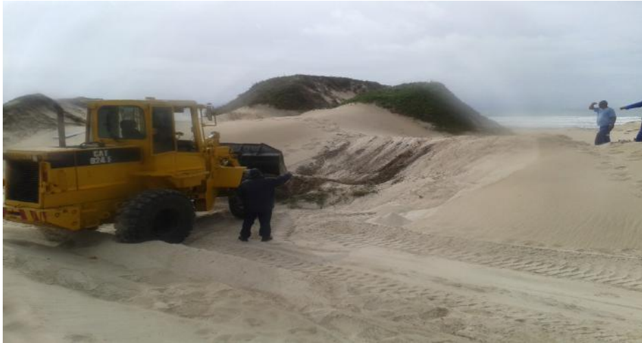
Front end loader clearing sludge off the dunes (Photo: D. Mentor 2017).
