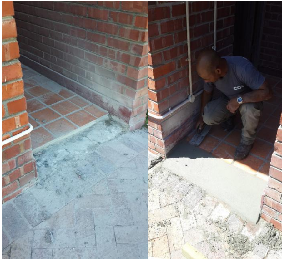
Henry Pheiffer fixing and building the wheel chair ramp (D. Mentor 2017).
